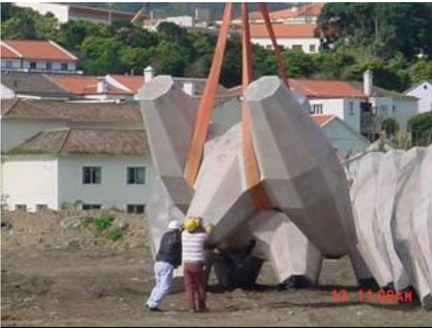
*35-ton CORE-Loc concrete armor unit.*
