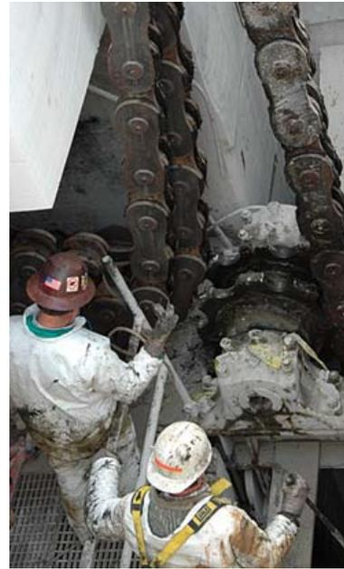
***January 7, 2006 - Crews from Midwest Foundation, Inc. remove two of the 25,000-pound liftgate chains from the west wall of the main chamber at Locks 27. The 50-year-old chains (four for each chamber) and other liftgate machinery are being removed and replaced as part of a rehabilitation project to the locks on the Chain of Rocks canal near Granite City, Illinois.***
