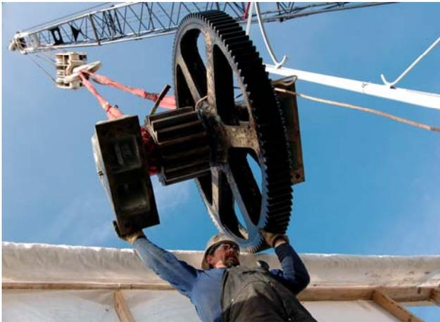
***February 6, 2006 – Millwright Wes Elliot steadies the countershaft and pinion gear as it is lowered into the machinery room in the west wall of the main chamber at Locks 27 near Granite City, Illinois. The refurbished countershaft and pinion gear is part of the \$13.46 million contract awarded to Midwest Foundation Corp. to rehabilitate the machinery and counterweights for both the auxiliary and main chambers at Locks 27.***
