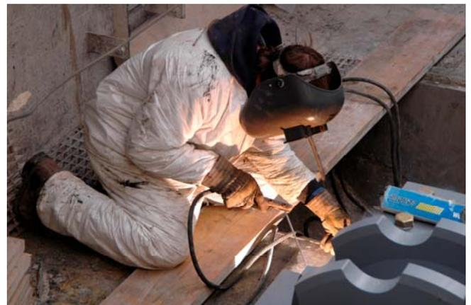
***February 6, 2006 – Curt Coleman welds a shear tab into place that supports the pillow block base for the idler sprocket. The idler sprocket supports the chain which is connected to the lift gate at one end and a counterweight at the other.***
